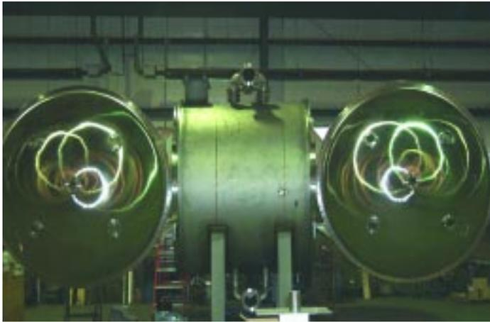
High-voltage charges in these stainless steel tanks produce ozone gas from oxygen for primary disinfection.
