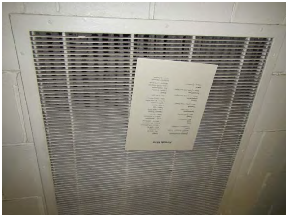
Wall-mounted return vent in (K213)-paper shows it drawing effectively
