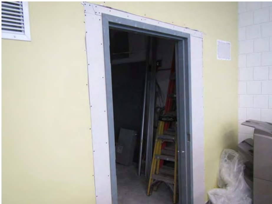
Elevator machine room renovations near Adjunct Faculty space (F202)
