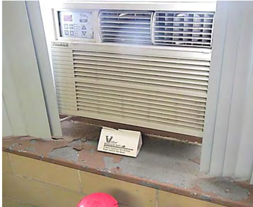
Peeling paint on windowsill
