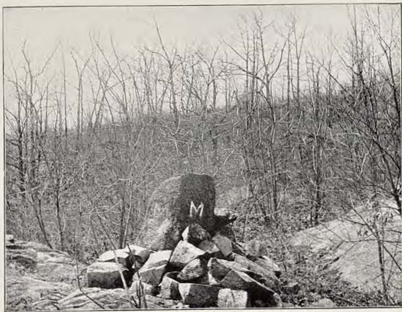
CORNER 1 (LOOKING SOUTHWESTERLY) — 1898.
