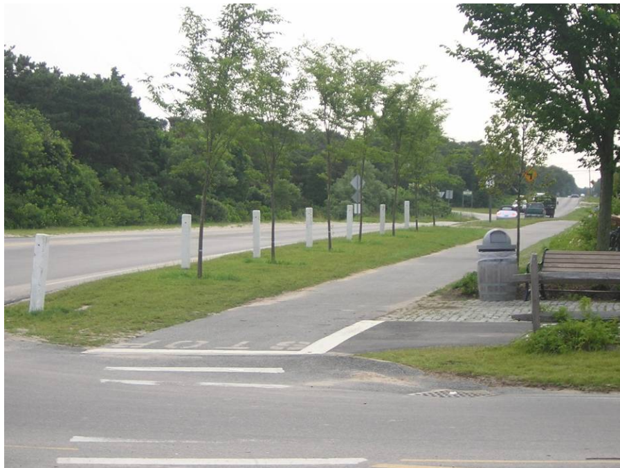
The DPW planted this line of trees along Milestone Road near the rotary.
