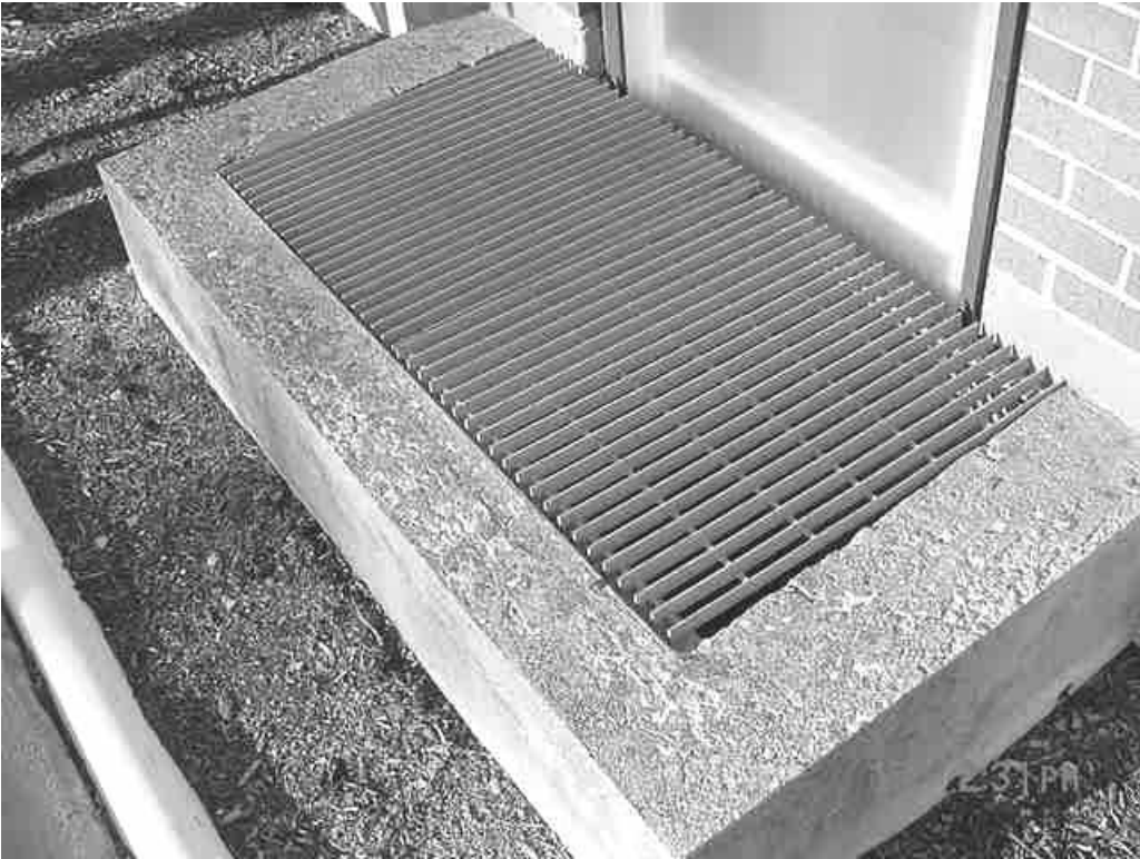
Subterranean Concrete-Lined Pit for Basement Univent Air Intake
