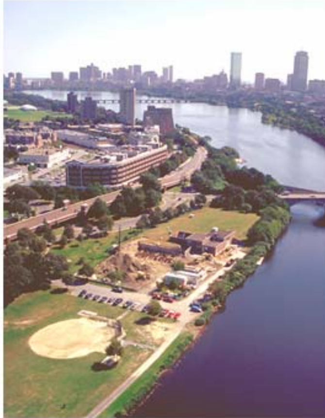
Figure 15: Aerial View of Cottage Farm Facility
