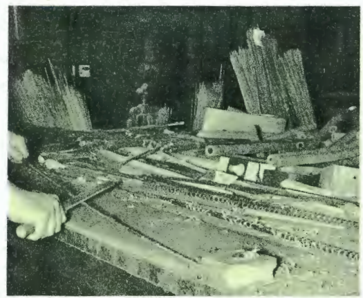
13 Removal of dry glue and wrapping.
