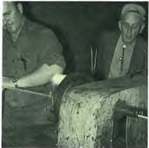
10 Glued section being wrapped — 200 lb. pressure.
