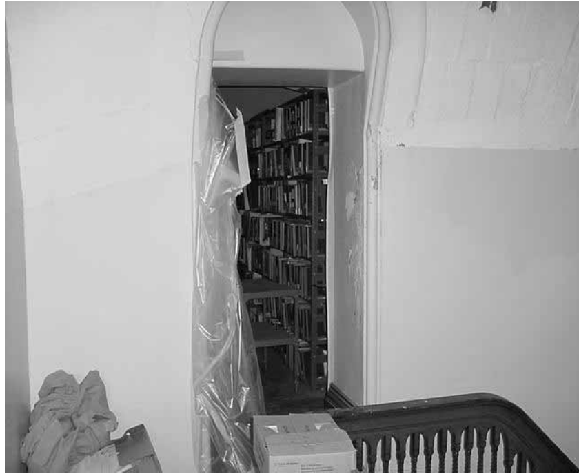
Book Storeroom off the Balcony above Clerk's Office Suspended Ceiling
