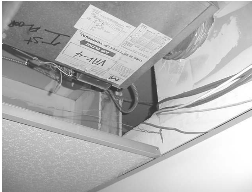
Typical Return Hole for 1 st Floor Office
