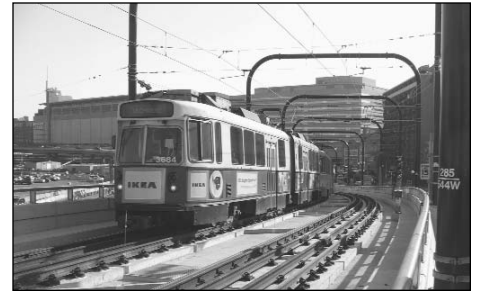
Green Line train on the new viaduct ramp
