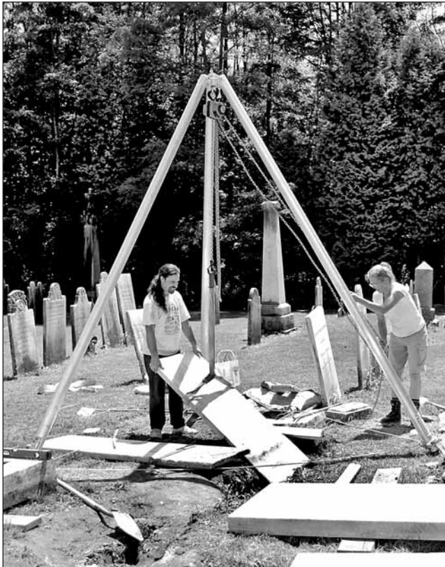
Ongoing grave stone repair work in Center Cemetery
