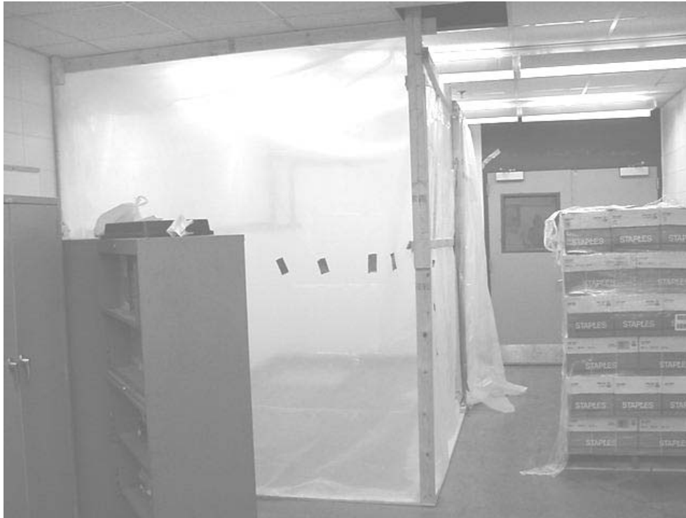
Containment Walls Constructed around Crawlspace Hatch in Room 123
