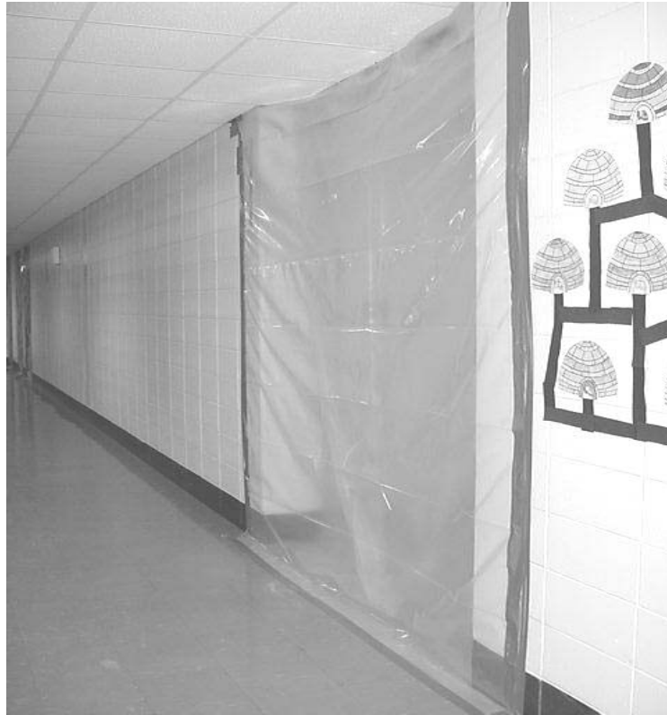
Plastic Poly Containment Wall, Note also Sealed on Interior Side
