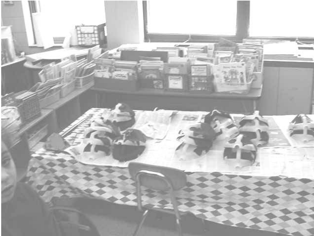
Classroom Univent Obstructed by Various Items
