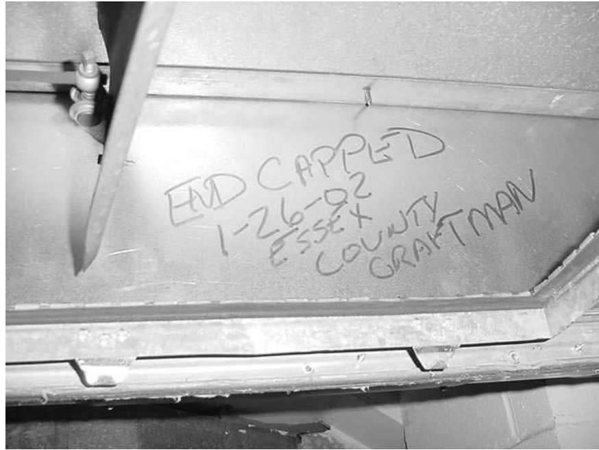
Sheet Metal Installed In Duct to Prevent Basement Draw
