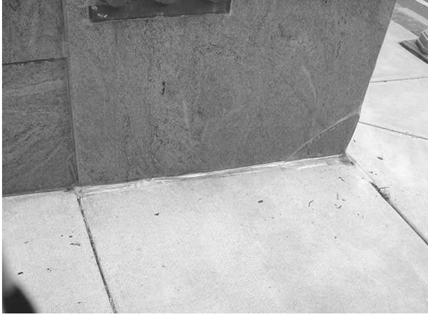
Sidewalk/Exterior Wall Seam Under Repair
