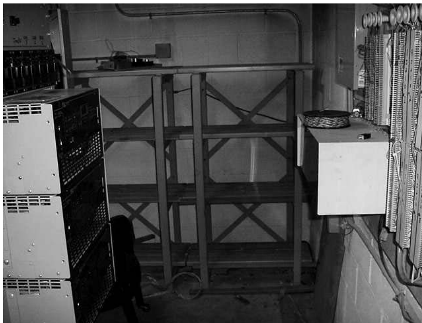
Batteries Were Removed From Basement
