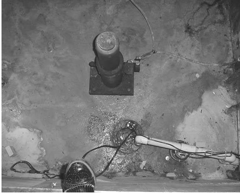
Floor Of Elevator Shaft Was Free Of Pooling Water
