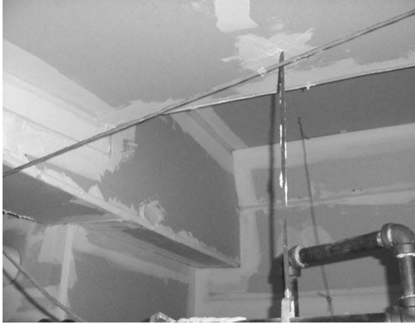
Replaced Gypsum Wallboard above 6 th Floor Elevator Lobby
