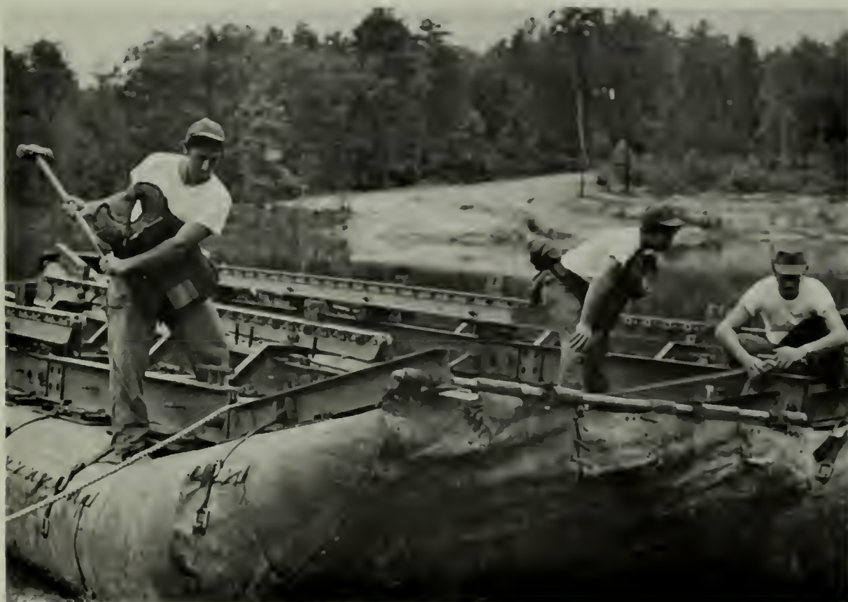
Personnel of 101 Engineer Battalion construct a pontoon bridge during Annual Training period
