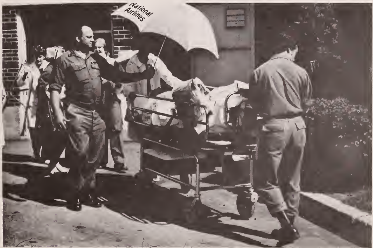
The transfer of patients from the old wing of the Faulkner Hospital to its newly constructed wing was a pleasant experience to many of the patients thanks to Massachusetts guardsmen.
