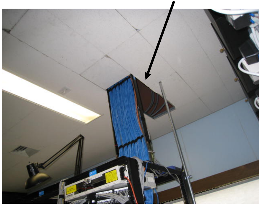
Space in Suspended Ceiling in Room 403C (arrow)
