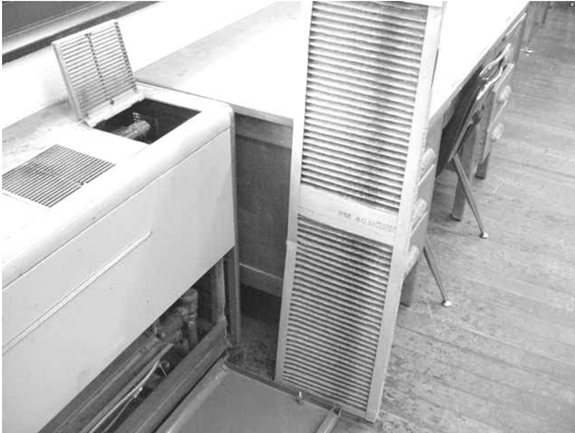
Soot Buildup on Univalent Filter as Indicated by Black Line across Filter Medium
