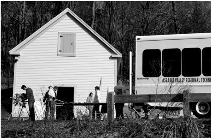
Assabet Valley carpentry students working at the new curatorial building.
