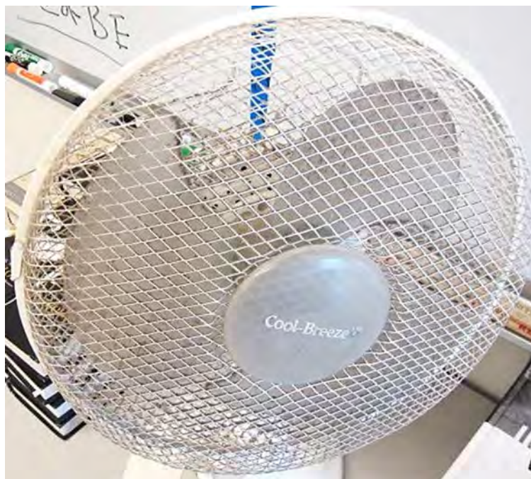
Accumulated dust/debris on fan blades in classroom
