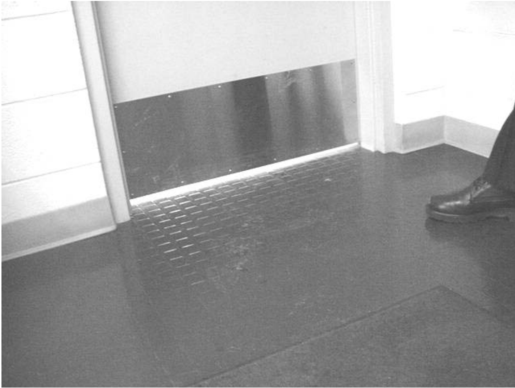
Space Beneath Stairway Door to Engine Bay
