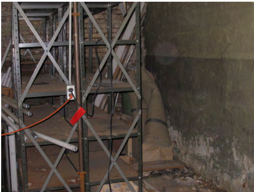
Rolled Up Carpet in Basement
