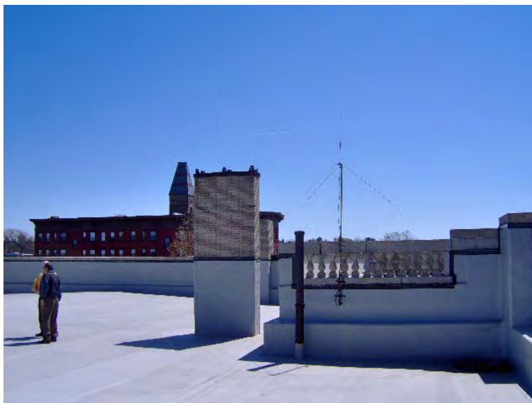
Likely Non-Motorized Exhaust Vent On Roof
