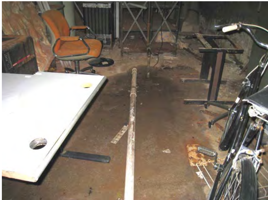
Pipe Terminus over Drain
