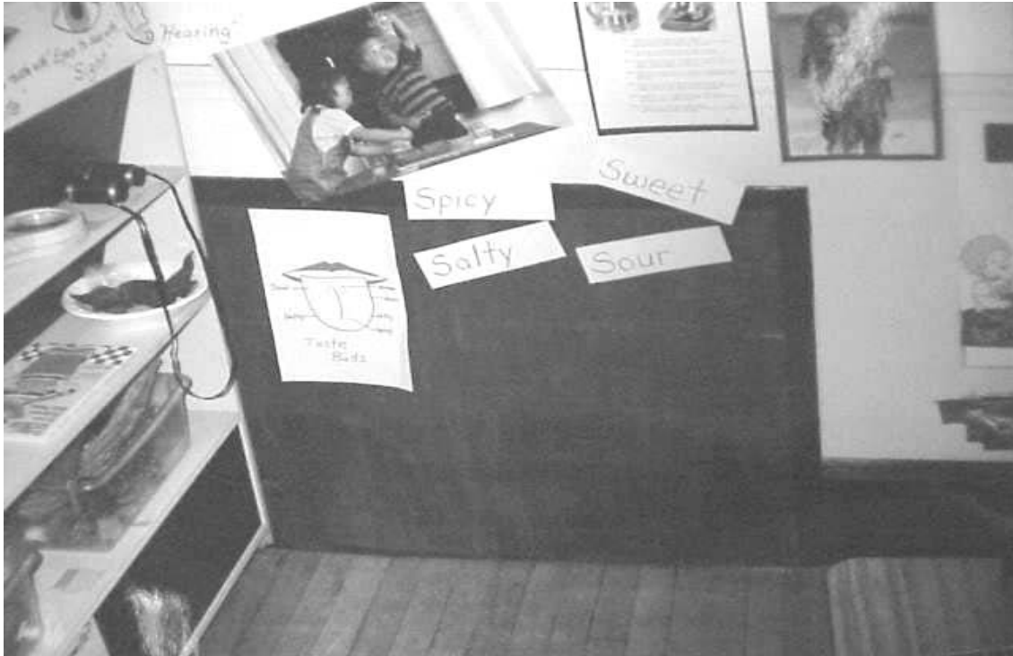
Sealed Natural/Gravity Feed Exhaust Vent Noted in Classroom
