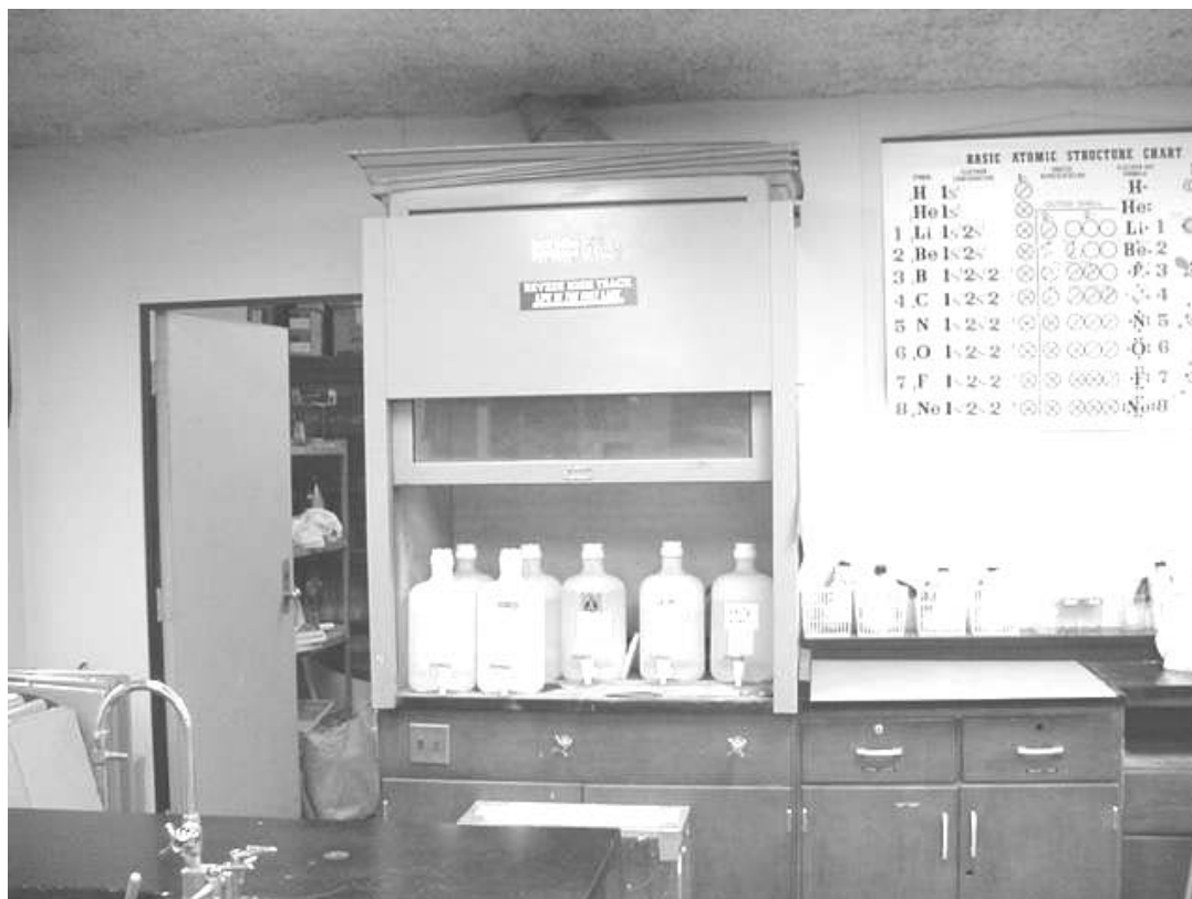
Chemicals Stored in Vent Hood, Note Vent Hood Not Operating During the Assessment
