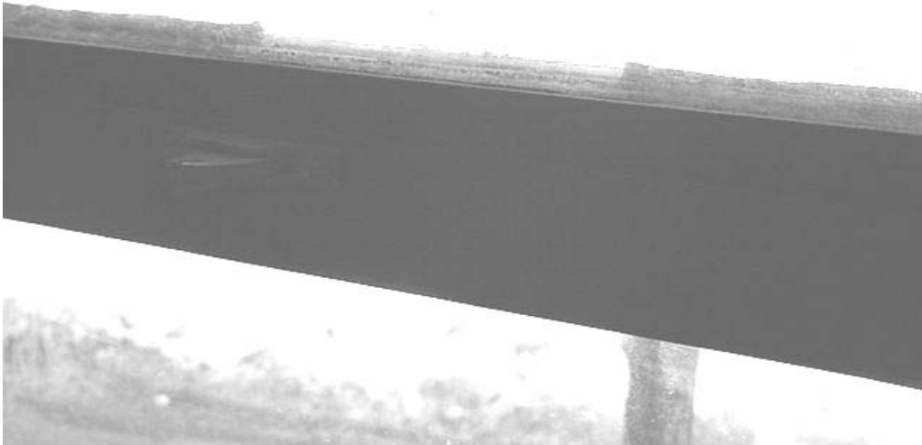
Missing/Damaged Window Caulking
