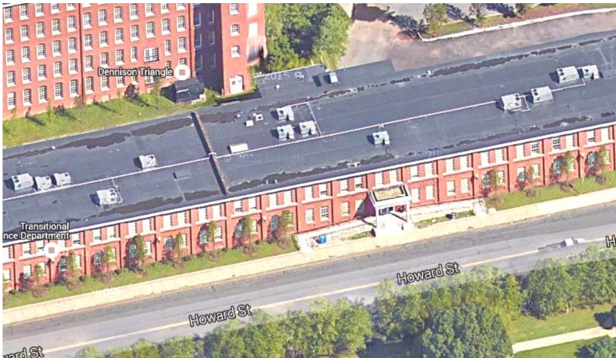
Rooftop air handling units
