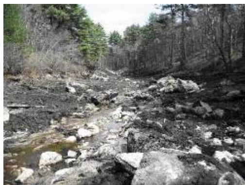
Sediment removed from former dam impoundment April 2010
