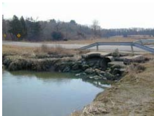
Old Metal Culvert
