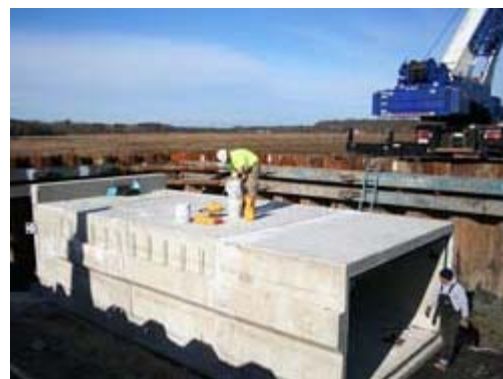
New Box Culvert
