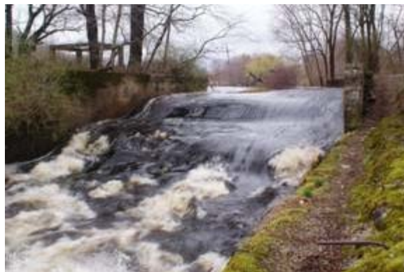
Flood flows passing over the State Hospital Dam this past March.
