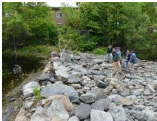
Emergency and temporary replacement for the Whittenton Mill Pond Dam.
