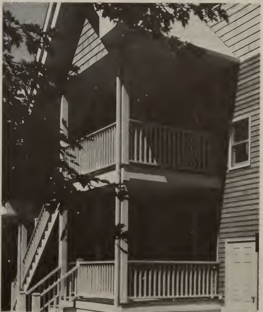
The woodframe building in Chelsea is part of a condominium development built through the HOP program. Now completely sold, the four-bedroom units were purchased with 7.9% MHFA loans on which the initial interest rate was reduced to 5% with HOP funds.
